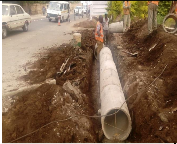
Laying of precast pipe culverts
