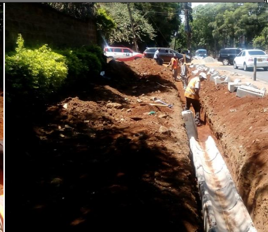
Laying and joining of IBDs
