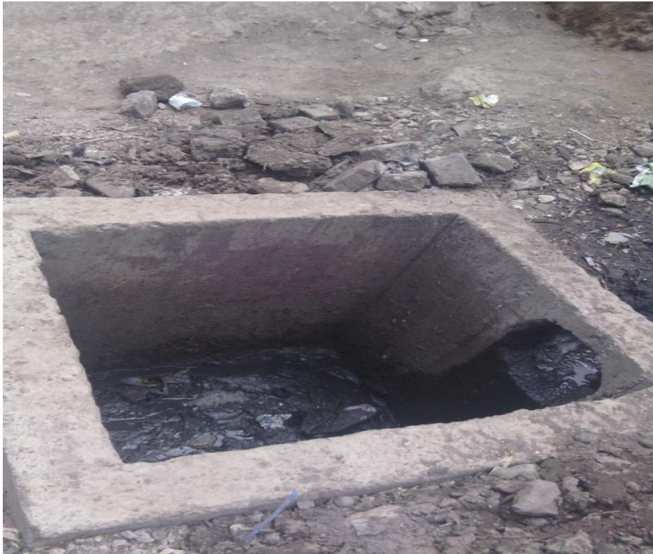
Figure 4.11: clogged up drain on BH-Road
