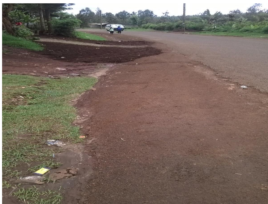
Figure 4. 3 section of the drain being blocked by heap of soil
