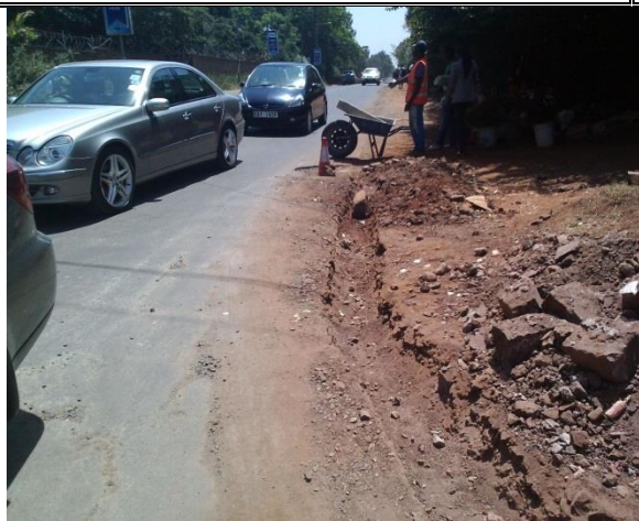
Excavation and levelling for kerbs installation
