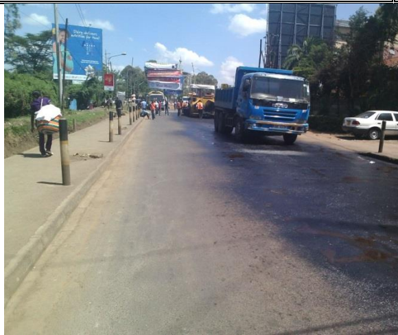
Spraying of k1-60 as tack coat.
