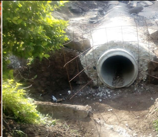
Reinforcing headwalls and wing walls
