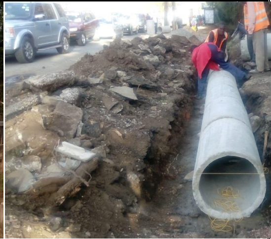
Laying and joining of precast pipe culverts
