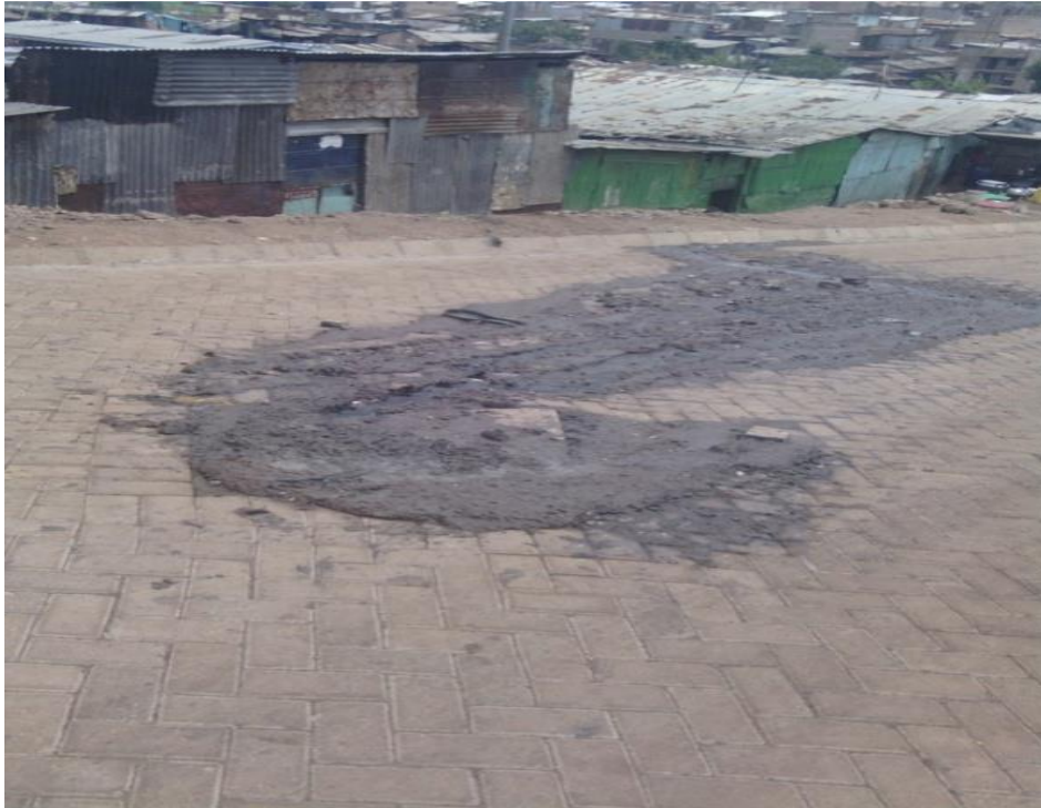
Figure 4.10: leaking sewer on BH road
