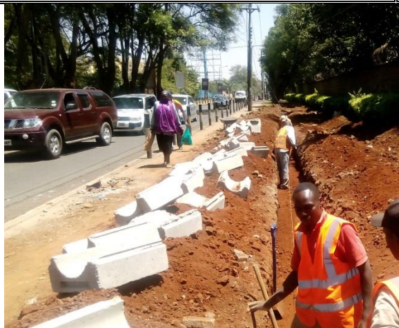
Excavation and levelling to IBDs
