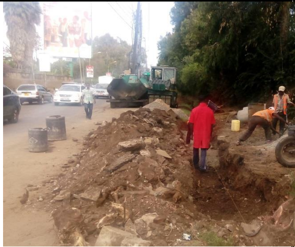
Excavation for culvert installation
